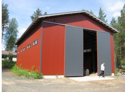
Figure 68. Toivakka heating plant, 0.7 MW (Jyrki Raitila)
