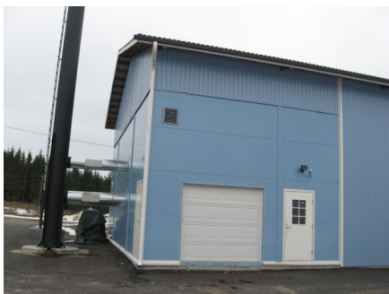
Figure 69. Joutsan Ekowatti plant (Jyrki Raitila)
